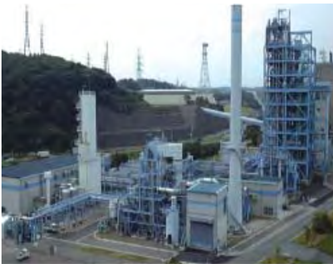
Photo 1 Pilot test facilities
